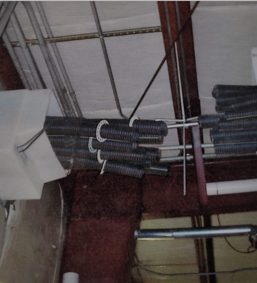
Connection of corrugated tubing
