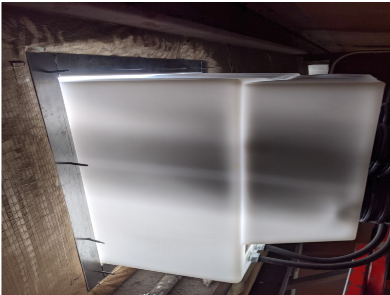
Inside installation Of Single Skin
