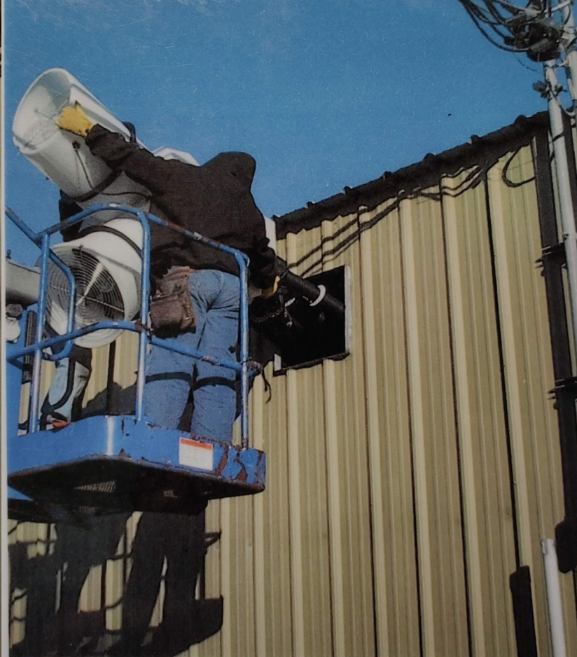
Installation of Unit
